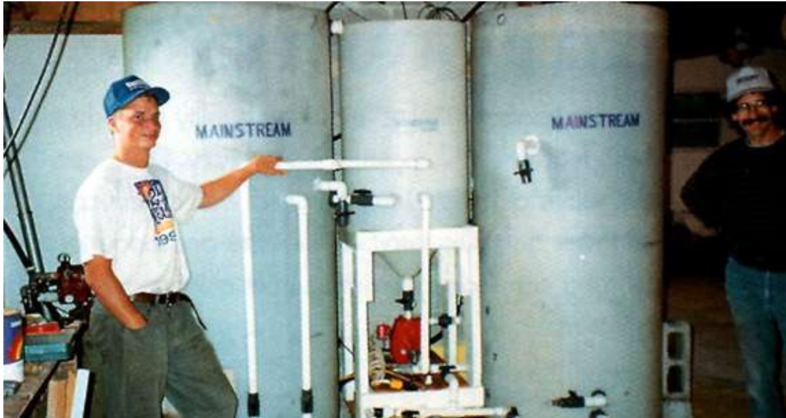
Photo 2. This initial prototype for surface water biological treatment system was installed for a farmer in December, 1993
