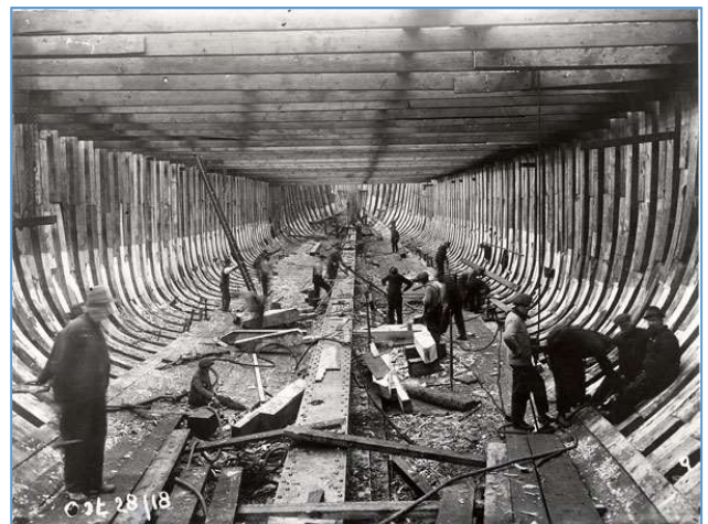
Figure 3. The photo shows builders at work in the interior of a boat. In the mid-19th century, shipbuilding was going full steam in New Brunswick. Each ship was built to its own specifications, depending on its intended use: hauling large cargos over the seas, speeding across the Atlantic, or carrying passengers. (Photo credit: Provincial archives of New Brunswick).
